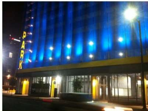
*ACTUAL PICTURE OF PARKING GARAGE*
